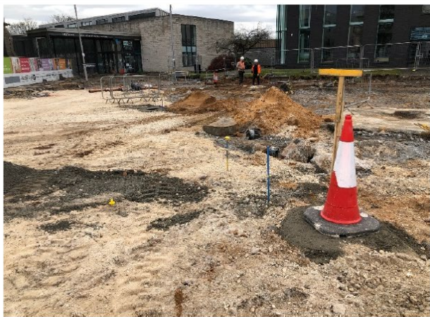
General progress photograph.
