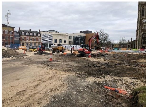
General progress – View North from Carlton St Vehicular gate.
