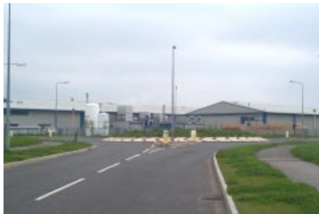
(left) - Modern galvanised steel columns used to illuminate a Primary Distributor road
