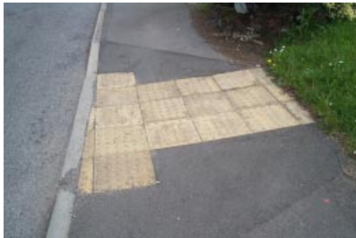
(right) - Pre cast concrete tactile paving blocks used as part of a dropped kerb
