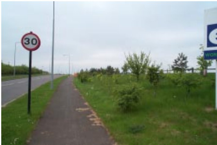
(left) - footway located behind grassed verge
