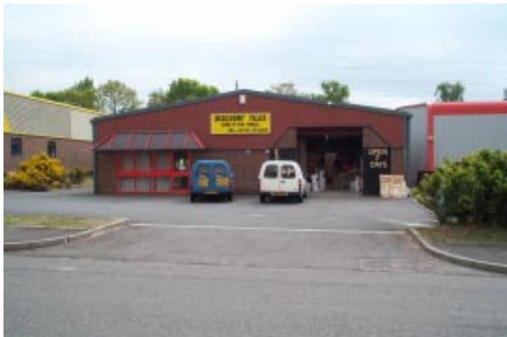
(left) - Junction serving a small industrial unit (Dropped kerbs & tactile paving must be provided)
