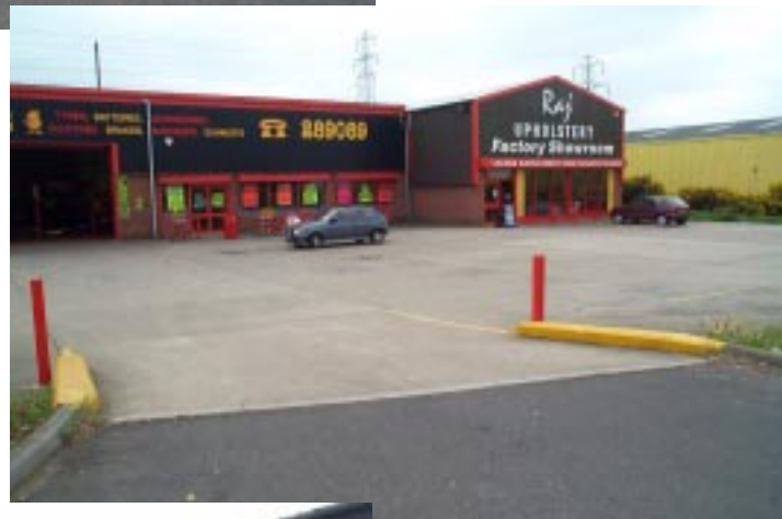
(right) - For a smaller site, again there is sufficient room within the site for manoeuvring, but HGV and car parking areas are not segregated
