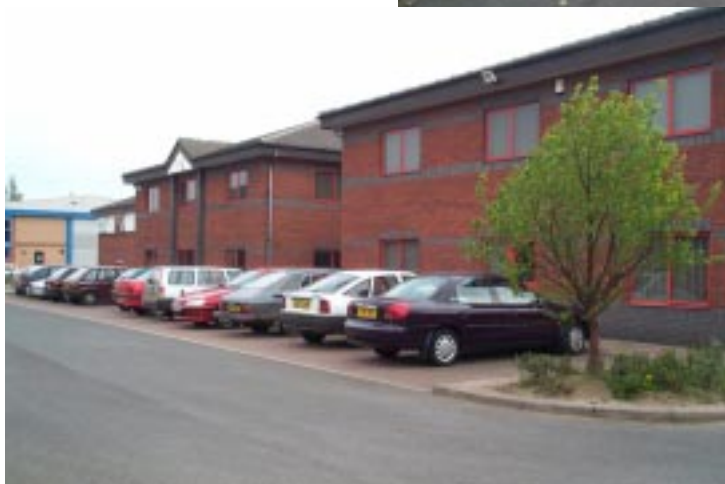
(left) - Parking suitable for office or high-tech types uses. Note the differing surface treatments of the isles and bays
