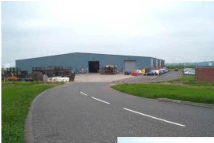
(left) - layout for a large factory site. there is sufficient room for HGVs to manoeuvre, and car parking is segregated from the loading area
